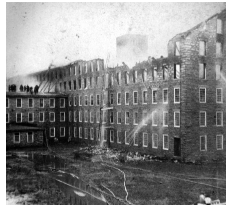
Figure 6. Granite Mill #1 with top two floors burnt out in 1874, showing that the fire was prevented from spreading to lower floors. Photo: (ATHM web).
