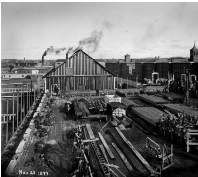
Figure 17. Reconstruction of Amoskeag Mill #4 and #5, 1899. This shows the last of the gable roofed mills in the Amoskeag Millyard being replaced with an updated mill that is wider than, but not as high as, the earlier mills. HABS copy photo.
