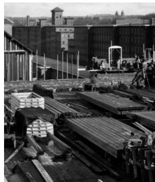
Figure 18. Detail of #17 showing the sawn and dressed heavy timber beams with cast iron seats already attached ready for erection. HABS copy photo. (Most copy photos from Manchester Historic
