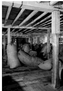
Figure 10. Interior showing beam-and-joist construction.
