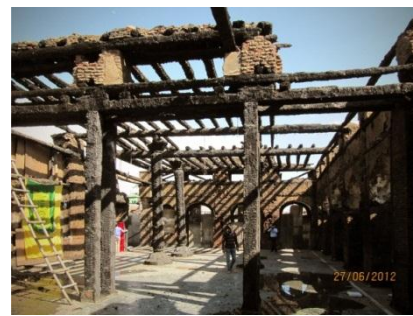
Figure 24. View of the fire and a view of the same space as in #24 after the fire destroyed the entire interior, leaving the heavy timbers charred but structurally sound. Needless to say, the loss of the artistic ornamental interior is a tragedy. The columns in the distance are two of those seen in the center of figure 23. Photo (center) Kashmir Monitor , (right) Hakim Sameer for INTACH .
