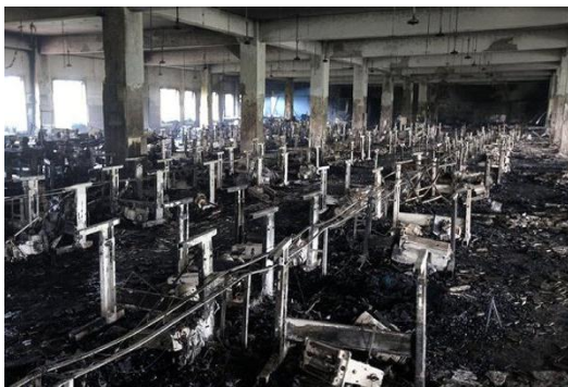
Figure 36. The Tazreen Fashions Factory, Bangladesh after the fire that killed 112 people. It appears from this image that the concrete structure was not even scorched, indicating that it was a flash fire that killed the people who could not get out. Photo Abir Abdullah/European Press Photo Agency.
