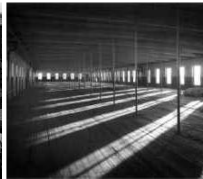
Figure 19. Interior of Stark Mill #3, Amoskeag Millyard, the day before it was demolished under "Urban Renewal". This shows the "slow-burning" heavy timber flat roof that was retrofitted onto this building after the earlier gable roof was removed. Photo © by the author.
