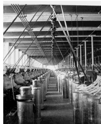
Figure 16. View of Carding Machine Room in the Jefferson Mill, Amoskeag Millyard. This view is of a mill ca. 1880, and shows beam and plank “ slow-burning ” construction. HABS copy photo.
