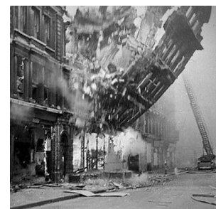
Figure 33. London Blitz fire in 1942 showing danger of outward falling walls. Image from Retro-naut.com
