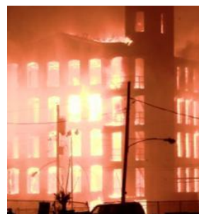
Figure 32. Abandoned Buck Hosiery Mill fire 9 April 2012. Effectiveness of fire cuts shown. From ABClocal.go.com
