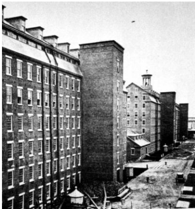
Figure 14. The ca. 1845 Bay State Mills in Lawrence MA. These mills, 9 stories including the two floor levels in the gambrel roof, may have been the tallest U.S. 19 th century mills ever constructed. They were demolished only 36 years after they were built. Late 19 th century mills were not so high in part because of inability to reach this height with hoses and ladders. In the 20 th century, the height limit was restricted to 65 feet (20 meters). Photo from (Langenbach 1981)
