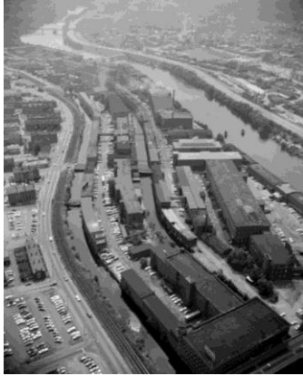
Figure 20. Aerial view of the Amoskeag Millyard in 1967 showing the canals on two levels. Photo taken in 1967 by the author for HABS.
