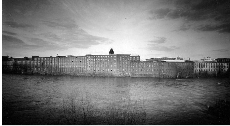
Figure 21. The southern end of the Amoskeag Millyard from across the Merrimack River. The original millyard had many separate “Lowell style” gable-roofed mills, but during the 2 nd half of the 19 th century, with improved firefighting equipment and full ‘slow-burning’ construction, the later buildings were joined together with internal firewalls. Photo © taken in 1968 by the author.
