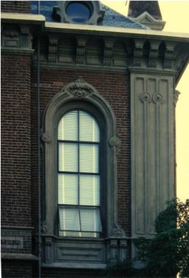
**Figure 6C:** Exterior of South Hall showing large ornamental cast iron corner bracket. The bond iron in the brick walls terminates at the large bosses.
