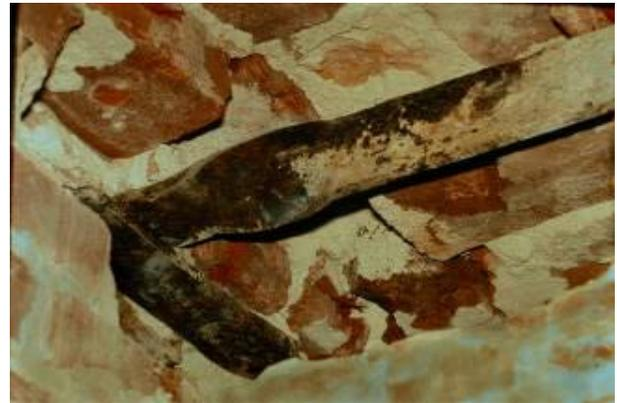
**Figure 6A:** Bond iron inside the brick exterior wall of South Hall exposed during construction work.
