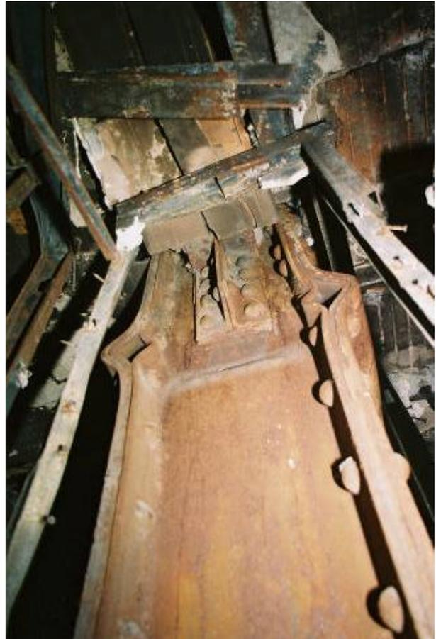
**Figure 3:** Buckled riveted steel column, 90 West Street
