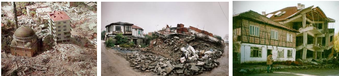
1999 EQ photos: Figure 10: Mosque and minaret still standing in Gölcük with collapsed RC buildings around it. (Al Jazeera) Figure 11: Hımsı house next to an entire row of collapsed RC buildings in Adapazari. Figure 12: Hımsı house next to destroyed RC building. (Adem Doğançün)
