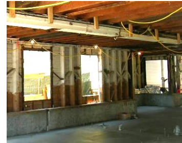
Figure 3: San Francisco 19 th century house with timber framing exposed.
