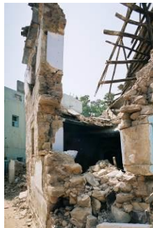
Figure 7: URM stone house in Bhuj after 2001 Gujarat earthquake. Figure 8: This man survived but his mother didn't, and he is cremating her, and holds her picture. Figure 9: Another view of the ruins of both stone houses and concrete houses in Bhuj.
