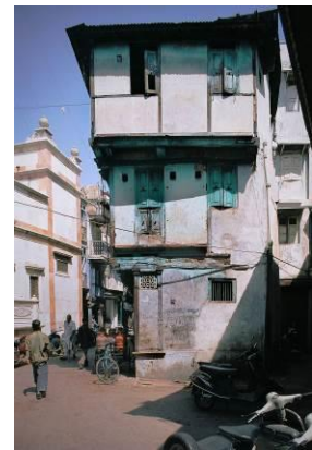
Figure 4: Hand cutting timber planks in Nepal, 2016. Figure 5: Colombage (Half-timber) house with almost no damage from the 2010 earthquake in Haiti. Figure 6: Half-timber 3 story house with almost no damage in 2001 earthquake in Ahmedabad, Gujarat.
