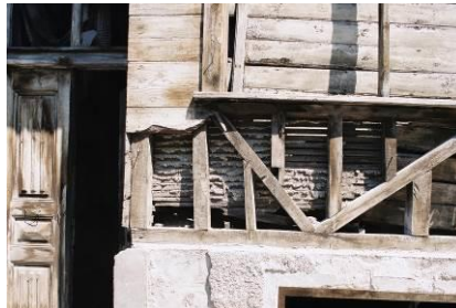
Figure 2: Stud framing typical in central Istanbul without infill masonry.
