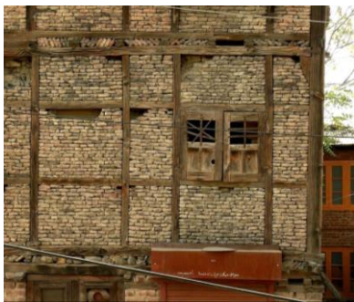
Figure 31: Srinagar, Kashmir dhajji structure without diagonals
