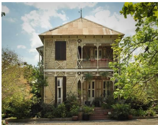
Figure 4: Hand cutting timber planks in Nepal, 2016. Figure 5: Colombage (Half-timber) house with almost no damage from the 2010 earthquake in Haiti. Figure 6: Half-timber 3 story house with almost no damage in 2001 earthquake in Ahmedabad, Gujarat.
