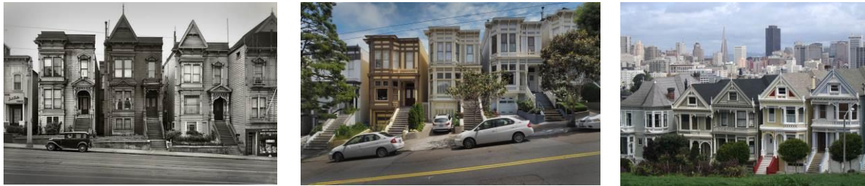
Figure 24, 25: San Francisco Victorians, 1940 (HABS), and today. 26: The “Painted Ladies” (B. Mittal)
