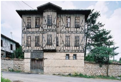
Figure 1: house with hımış on the 1 st and 2 nd floors, and hatil on the ground floor in Safranbolu.
