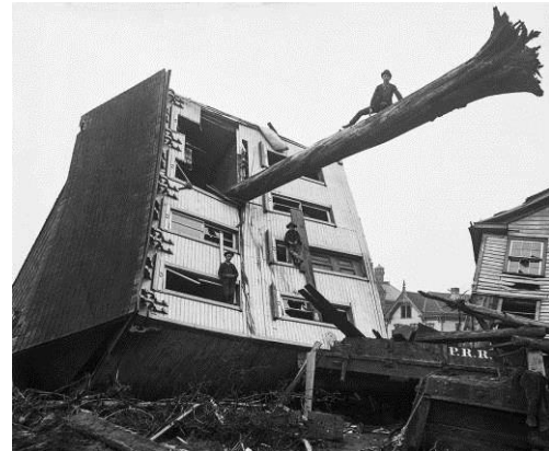
Figure 29: Wooden houses on Howard street, only one of which remains still centered on its foundation. Most interesting is that they managed to hold the line against the fire with these houses facing ones burning. (The Atlantic, 4/11/16) Figure 30: John Shultz House after the 1889 Johnstown dam burst, a remarkable visual testament to the resilience of 19 th century stud frame construction. (Bettmann/Getty Images)
