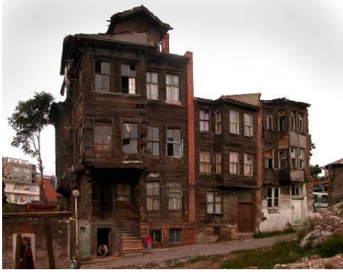
Figure 17: Houses with firewalls.
