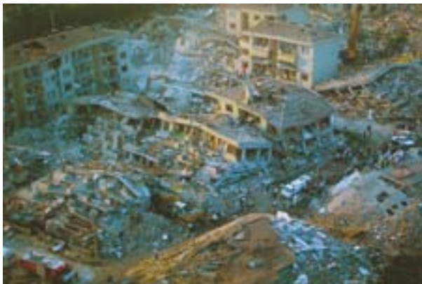
A row of collapsed buildings in Golcuk, Turkey, after the 1999 earthquake. © courtesy of United Nations
