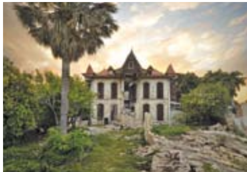
The Villa Castel Fleuri, which was constructed with walls of brick and rubble stone, was still standing after the 2010 Haiti earthquake. © Randolph Langenbach
