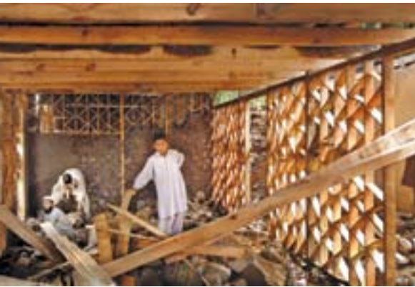
New dhajji construction in Thub, Pakistan. © Maggie Stephenson/UN-Habitat
