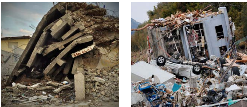
Figure 7. Left: Pancake collapse of a reinforced concrete building that was located in the Gingerbread District of Port-au-Prince. Right: As a remarkable example of the inherent strength and resilience of a well-constructed reinforced concrete building, this one in Rikuzentakata, Japan was swept onto its side and carried upstream by the March 10, 2011 earthquake and tsunami without being crushed or collapsed (AFP/Getty).
