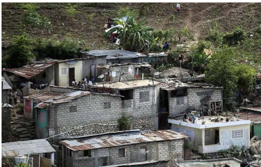
Figure 9. View of 4 Carrefour Feuilles area bidonville, close to the city center, Port-au-Prince showing the unsophisticated rough construction of informal settlement dwellings, with incomplete frames, round-rock rubble stone retaining walls, and unreinforced concrete block construction – that nevertheless did not collapse (Source: Carlos Barria-Reuters).
