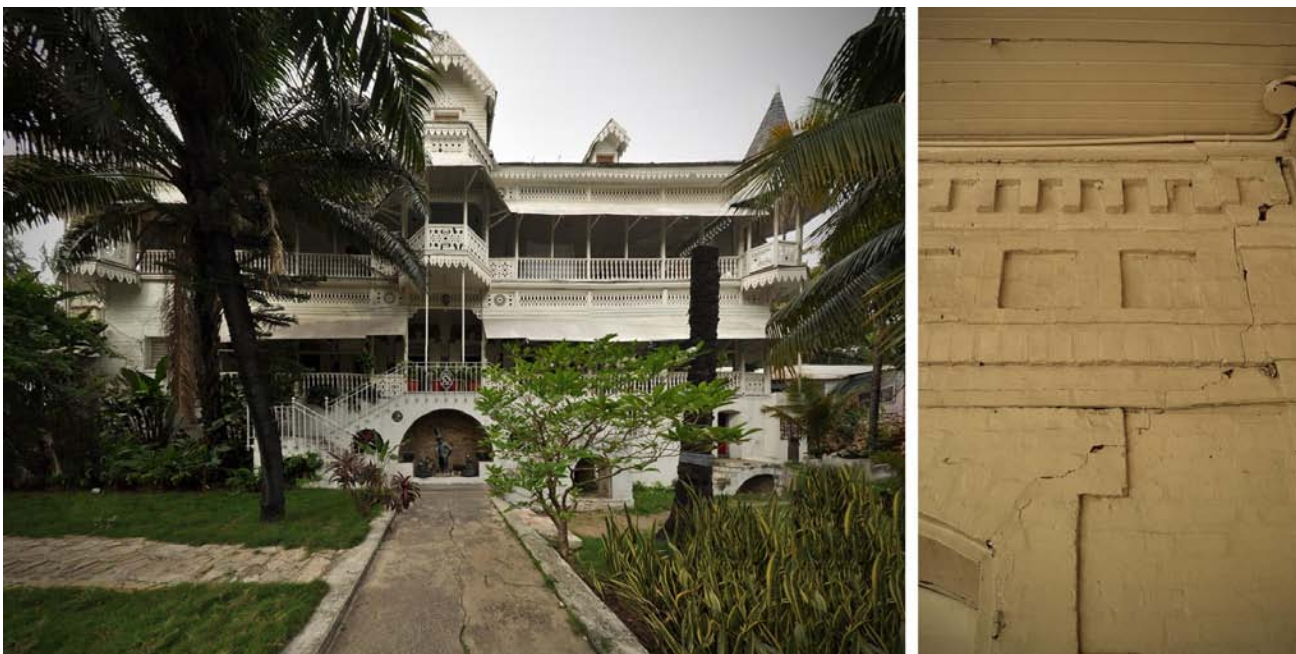
Figure 3. The unreinforced brick masonry Hotel Oloffson, Port-au-Prince after the earthquake.
