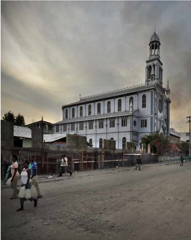
13. Saint Louis de Gonzague Chapel ca. 1890 in central Port-au-Prince showing external lightweight steel frame on masonry walls.
