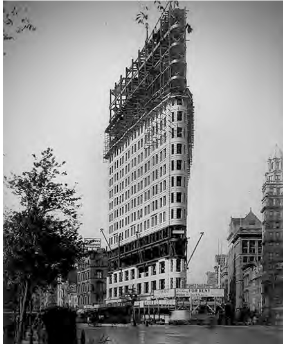
Fig. 3.12 Flatiron Building in New York City under construction in 1902 showing the heavy stone masonry façade resting on the steel frame. The upper walls were constructed separately probably to ensure the weight is bearing on the frame rather than the lower masonry walls. U.S. Library of Congress Photograph
