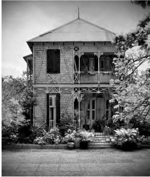
Fig. 3.6 A single family middle class house of colombage timber frame with single layer infill masonry construction near downtown Port-au-Prince photographed after the 2010 earthquake. This house was in the heart of the damage district with collapsed reinforced concrete buildings nearby. Photograph by © Randolph Langenbach
