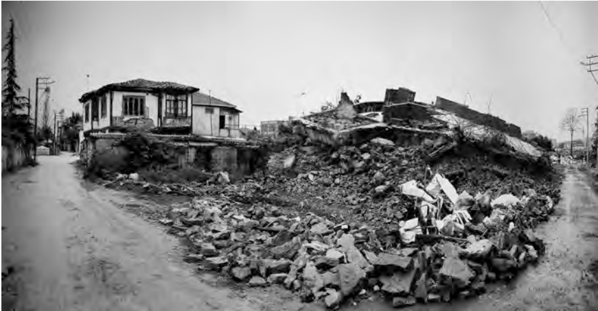
Fig. 3.1 A traditional humuş construction house still standing next to a row as far as one can see of reinforced concrete apartment buildings in Adapazari, Turkey after the 1999 Kocaeli earthquake. Photograph by © Randolph Langenbach
