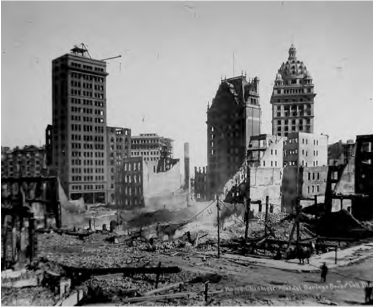
Fig. 3.13 View of San Francisco after the 1906 earthquake and fire. The three tall buildings visible in this view were burned out by the fire that followed the earthquake, but all three were in good enough condition despite this to be repaired, and they are still extant today. Photograph courtesy Bancroft Library, U.C.Berkeley
