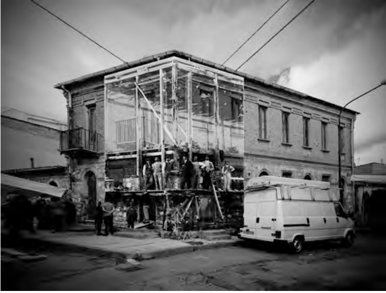
Fig. 3.7 An early 20th century building in Mileto, Calabria, Italy constructed with a baraccata timber frame embedded on the inside face of the wall, with a photo of it taken during its construction. Photo courtesy of the owner
