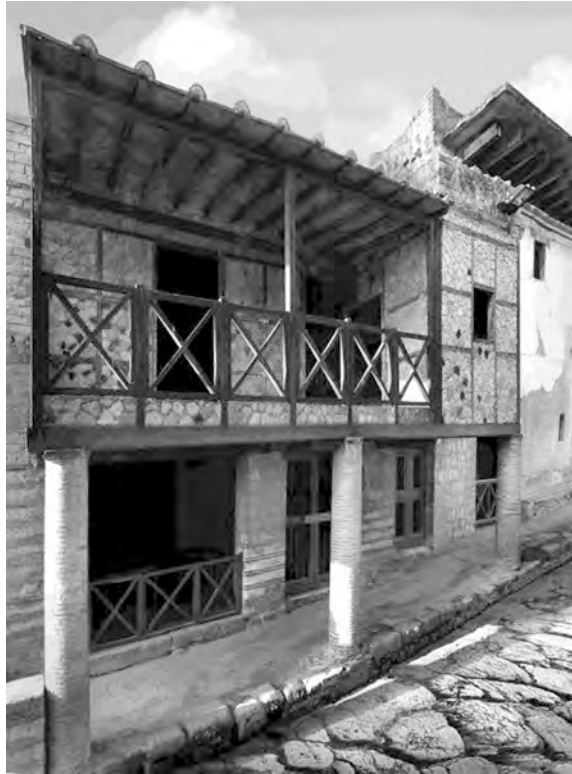
Fig. 3.5 A building in the ancient Roman town of Herculaneum uncovered after having been buried in the eruption of Vesuvius showing an example of timber frame with masonry infill that is thought to have been called Opus Craticium. Photograph by © Randolph Langenbach
