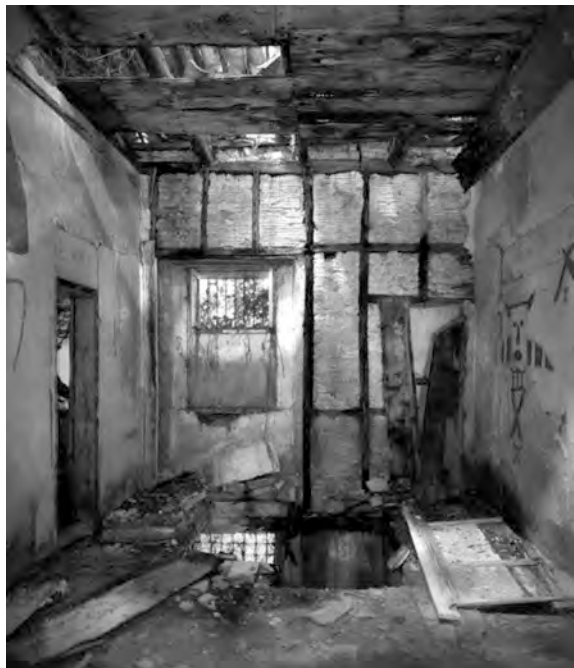
Fig. 3.10 Interior elevation view of the same wall as shown in Fig. 3.9 of the embedded casa baraccata framework in the Bishop's House in Mileto, Calabria, Italy. Photograph by © Randolph Langenbach
