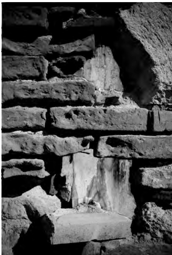
Fig. 3.8 A vertical column of the timber frame in the building in Fig. 3.7 showing through holes in the brickwork. Photograph by © Randolph Langenbach
