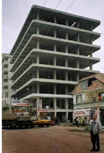
20. Building under construction in Gölcük, Turkey shown after the 1999 earthquake. Because the masonry infill walls had not yet been installed, frame action was able to occur, and thus the building was not collapsed by the earthquake.
