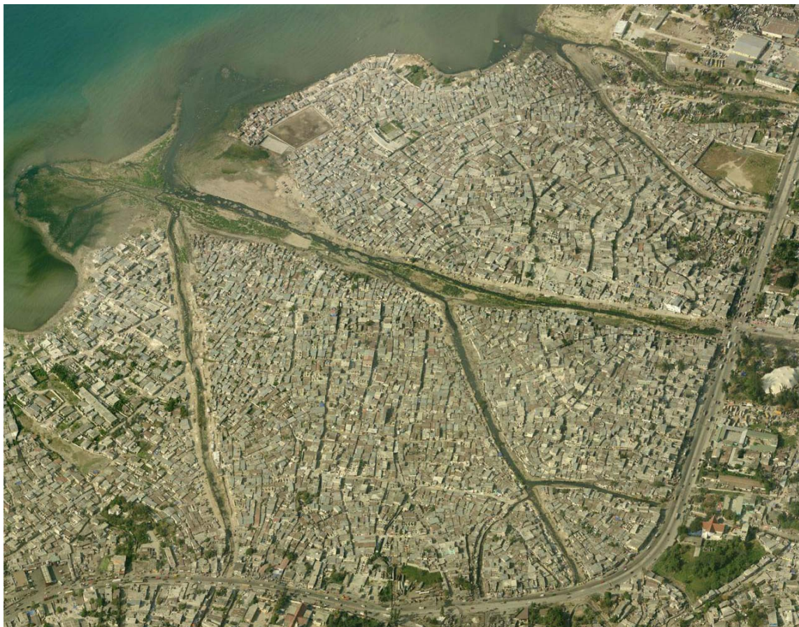
15a. Aerial view of Cité Éternelle, located on a combination of fill and an alluvial fan in central Port-au-Prince. Images © Pictometry. Mosaic of images into a single view by Randolph Langenbach
