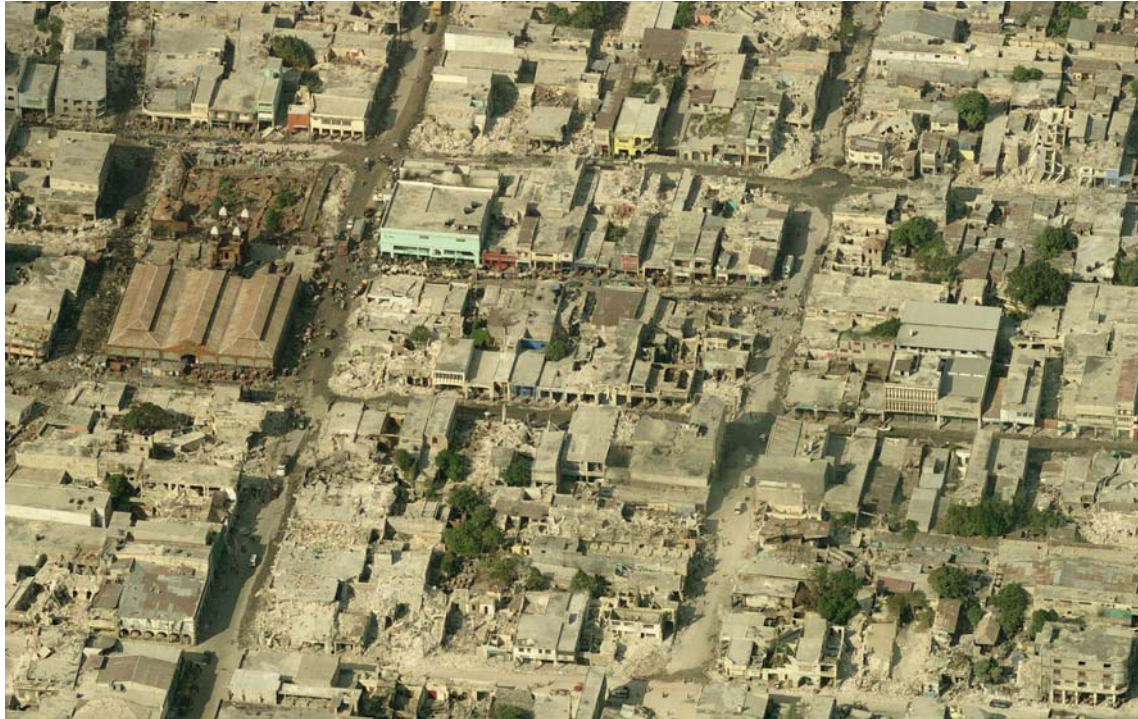
3. A detail from a Pictometry oblique aerial view of central Port-au-Prince one week after the earthquake. The collapsed unfinished building in Figure 1 is visible in the upper left. Photo © Pictometry International Corp.
