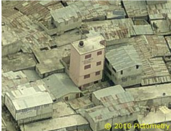
15b. Typical detail of Cité Eternal showing that two story buildings with one four story building – most of reinforced concrete. © Pictometry
