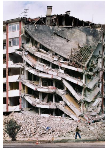
21. Building in Gölcük close to the one shown in Fig. 17 collapsed by 1999 earthquake. The heavy masonry infill walls together with open (soft) ground floors were often contributors to such collapses.
