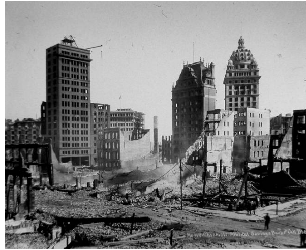
18. View of San Francisco after the 1906 earthquake and fire. The three tall buildings visible in this view were burned out by the fire that followed the earthquake, but all three were in good enough condition despite this to be repaired, and they are still extant today.
