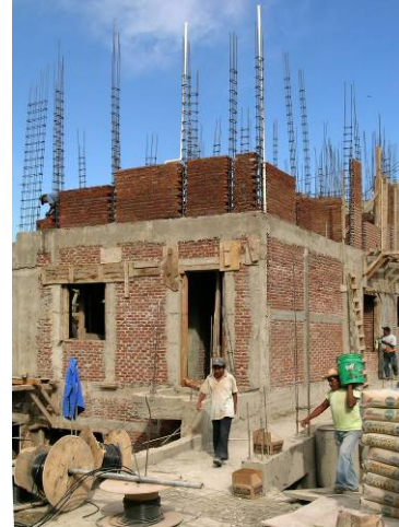
25. left , View of 4 Carrefour Feuilles area bidonville , close to the city center, Port-au-Prince. Source: Carlos Barria-Reuters Right , Confined masonry construction photographed in Zihujatanejo, Mexico.
