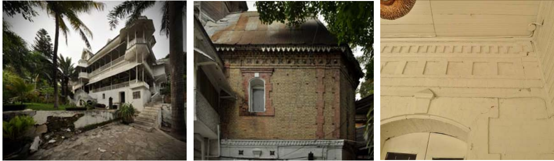
9. The unreinforced brick masonry Hotel Oloffson, Port-au-Prince after the earthquake. © Randolph Langenbach
