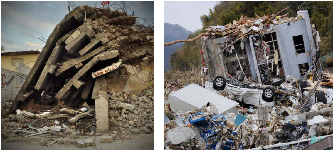
13. left : Pancake collapse of a reinforced concrete building on east (away from epicenter) side of Port-au-Prince. Pancake collapses of the heavy floors of multi-story RC buildings are particularly lethal and make it hard to extract the survivors. © Randolph Langenbach . Right : Reinforce concrete building in Rikuzentakata, Japan swept onto its side and carried upstream by the March 10, 2011 earthquake and tsunami. AFP/Getty
