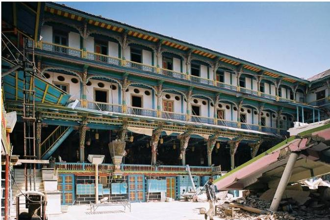
Fig. 4 This building in the Bhuj branch of the Ahmedabad-based Swaminarayan Temple is located in the heart of the walled city of Bhuj, yet it survived almost undamaged, while the modern concrete pavilion seen on the right collapsed. The construction is of timber frame with masonry infill, like that otherwise common in Ahmedabad, but rare in Bhuj.
