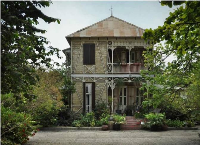
Fig. 10 A late 19<sup>th</sup> century house of *colombage* construction in Port-au-Prince after the 2010 earthquake. This house, despite its age, suffered only minor damage. *Colombage* is the French word for timber frame with infill masonry construction, similar to that found in Turkey, as well as in India in Srinagar and Ahmedabad.
