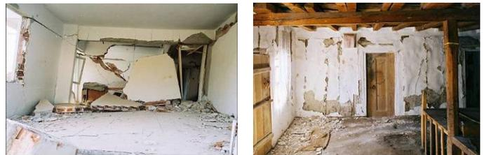
Fig 7 left: A view of a collapsed infill masonry wall in a reinforced concrete building in Gölçük, Turkey after the 1<sup>st</sup> 1999 earthquake, showing how the brittle masonry wall can collapse out of the concrete frame soon after it begins to crack when the frame deforms from the earthquake forces. right: A view of a *humus* construction wall showing how the timber frame has held the masonry panels in place for the duration of the earthquake, despite the shedding of the plaster surface.
