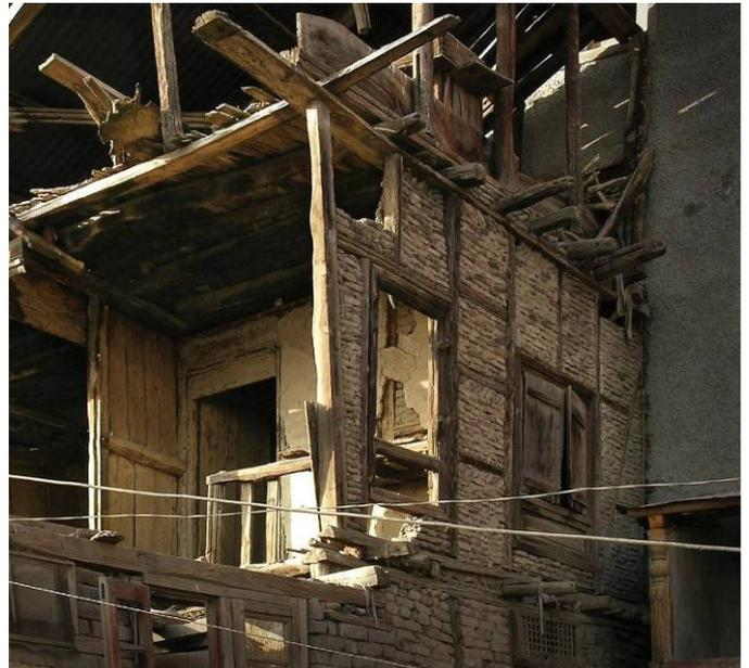
Fig. 2 Detail of *dhajji dewari* construction in a building under demolition in Srinagar, showing the timber frame, with the single-layer brick masonry infill. The walls are thin and light, when compared to bearing wall masonry. Notice how the floor joists are sandwiched between timbers at the floor level. This gives a strong friction connection between the floor diaphragms and the walls.
