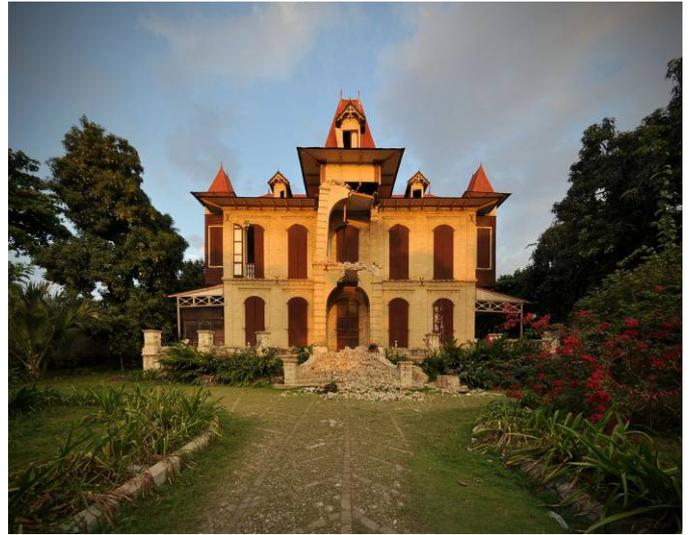
Fig 11 A late 19<sup>th</sup> century house in Port-au-Prince after the 2010 earthquake. The construction of the masonry walls in this house is a combination of brick and rubble stone. Despite the use of extensive internal sections of rubble stone, the house remained standing, although extensively damaged – thus showing a better performance than at least 40% of the reinforced concrete buildings in Port-au-Prince, which collapsed.
