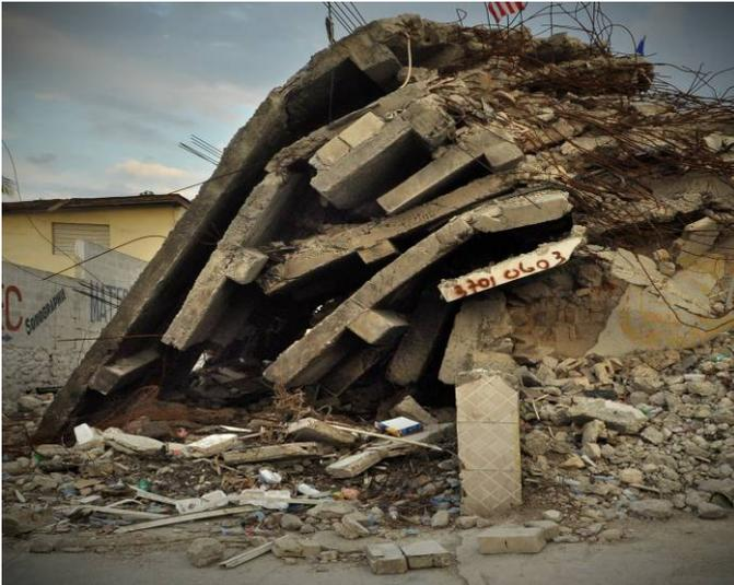
Fig.9 Remains of a collapsed multi-storey building in Port-au-Prince Haiti after the 2010 earthquake that devastated the city. The pancake collapse of reinforced concrete buildings is usually lethal to most of the occupants, and because of the strength of the concrete floor slabs, the finding and extraction of the survivors in time is exceedingly difficult.
