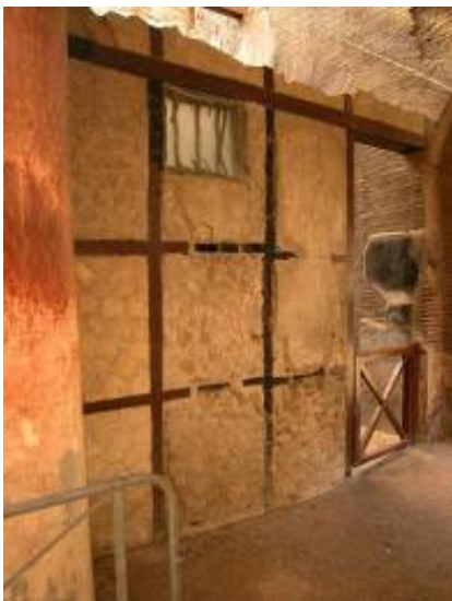
Fig. 12. Ancient Roman interior wall of Opus Craticium construction excavated in Herculaneum, Italy.
