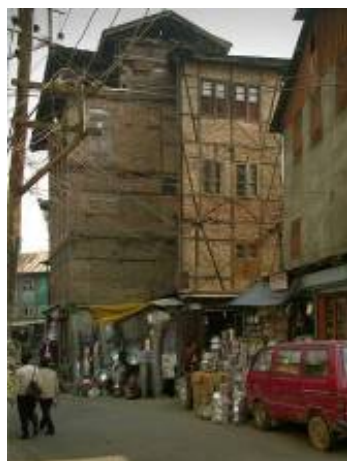
Fig. 9. Buildings in Srinagar, Kashmir. The building on the left is of taq construction, and on the right is of dhajji dewari construction.
