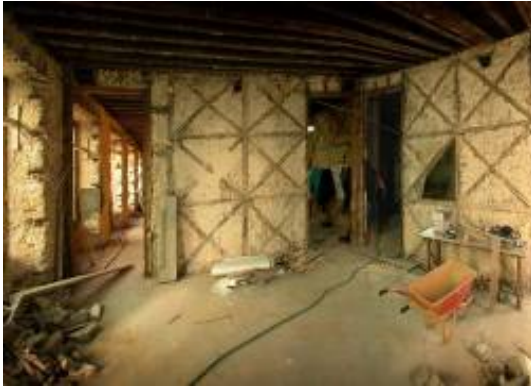
Fig. 16. 18th century building in central Lisbon showing 'Pombalino gaiola' construction, 2003.
