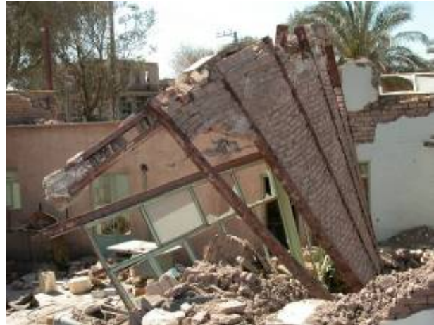
Fig. 4. Ruins from the 2003 Bam earthquake showing the steel and fired brick masonry jack-arch construction used for floors and roofs in Bam that were strong in themselves, but incompatibly rigid for the Khesht (unfired adobe) walls.
