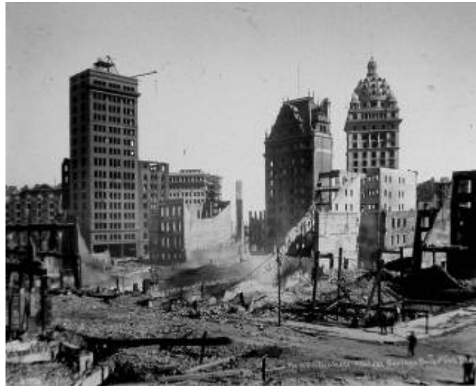
Fig. 22. View of San Francisco after the 1906 earthquake and fire. The three tall buildings visible in this view were burned out by the fire that followed the earthquake, but all three were in good enough condition despite this to be repaired, and they are still extant today.
