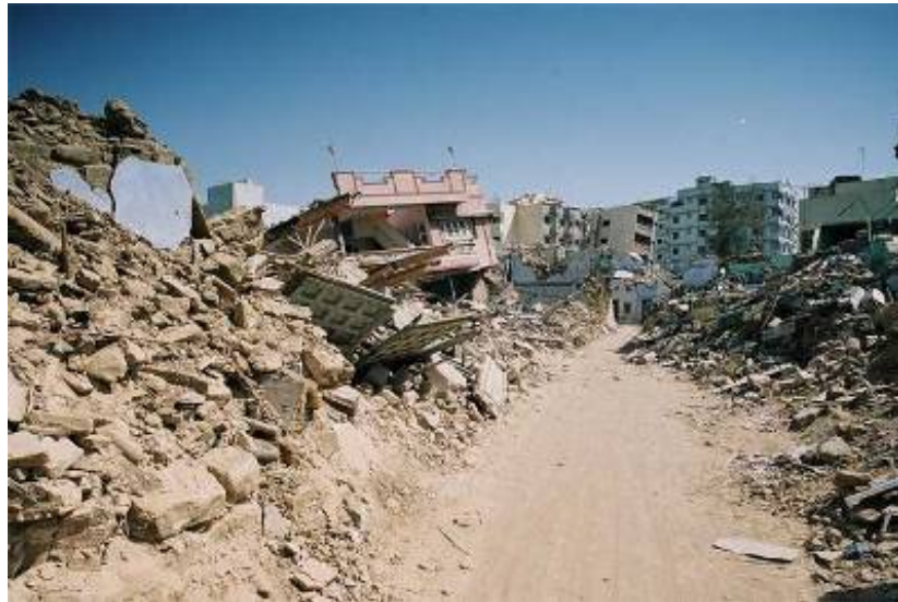
Fig. 15. In Bhuj, Gujarat, ruins of unreinforced rubble-stone buildings that collapsed during the 2001 earthquake. Unlike in Ahmedabad, much of the historic center of Bhuj, which lacked timber-laced construction, was destroyed.
