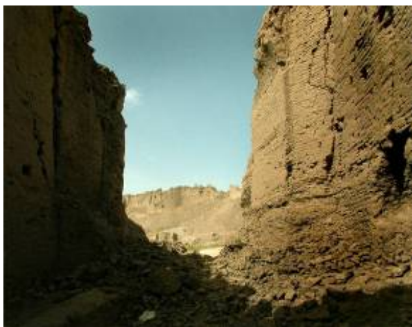
Fig.30. View from the Shahrbast Wall looking towards the ruins of the inner citadel of the Arg e-Bam. These towering walls, gnarled by time, were largely unaffected by the earthquake.
