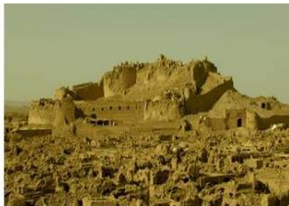
Fig. 2. The Arg-e-Bam, exactly the same view after the earthquake.
