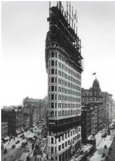
Fig. 21. Flatiron Building in New York City under construction in 1902 showing the heavy stone masonry façade resting on the steel frame. The upper walls are constructed separately probably to ensure the weight is bearing on the frame rather than the lower masonry walls.
