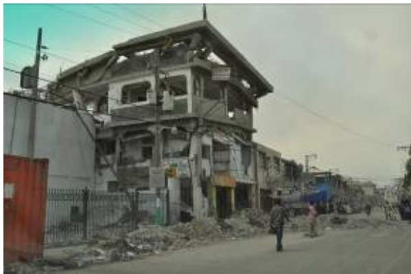
Fig. 19. Reinforced concrete building in central Port-au-Prince nearly collapsed by the 2010 Haiti earthquake.
