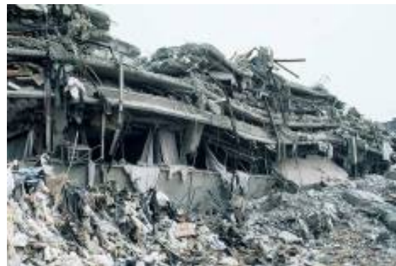
Fig. 8. The Juarez Hospital collapsed by the 1985 Mexico City earthquake.
