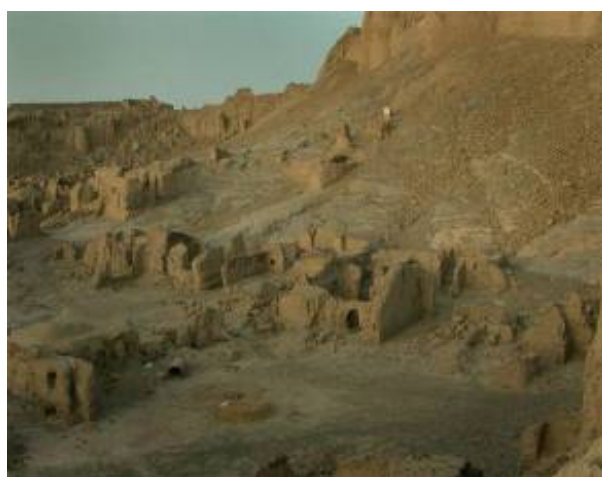
Fig. 31. The unrestored ruins in the Konari neighborhood of the Arg -e-Bam after the earthquake. Although abandoned and untouched for more than 150 years, these structures survived the earthquake with comparatively little damage.
