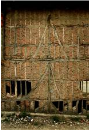
Fig. 5. Partially demolished house in Gölcük, Turkey at the time of the earthquake showing the single brick wythe thickness of typical hımış wall. The building had been abandoned for many years prior to the earthquake.
