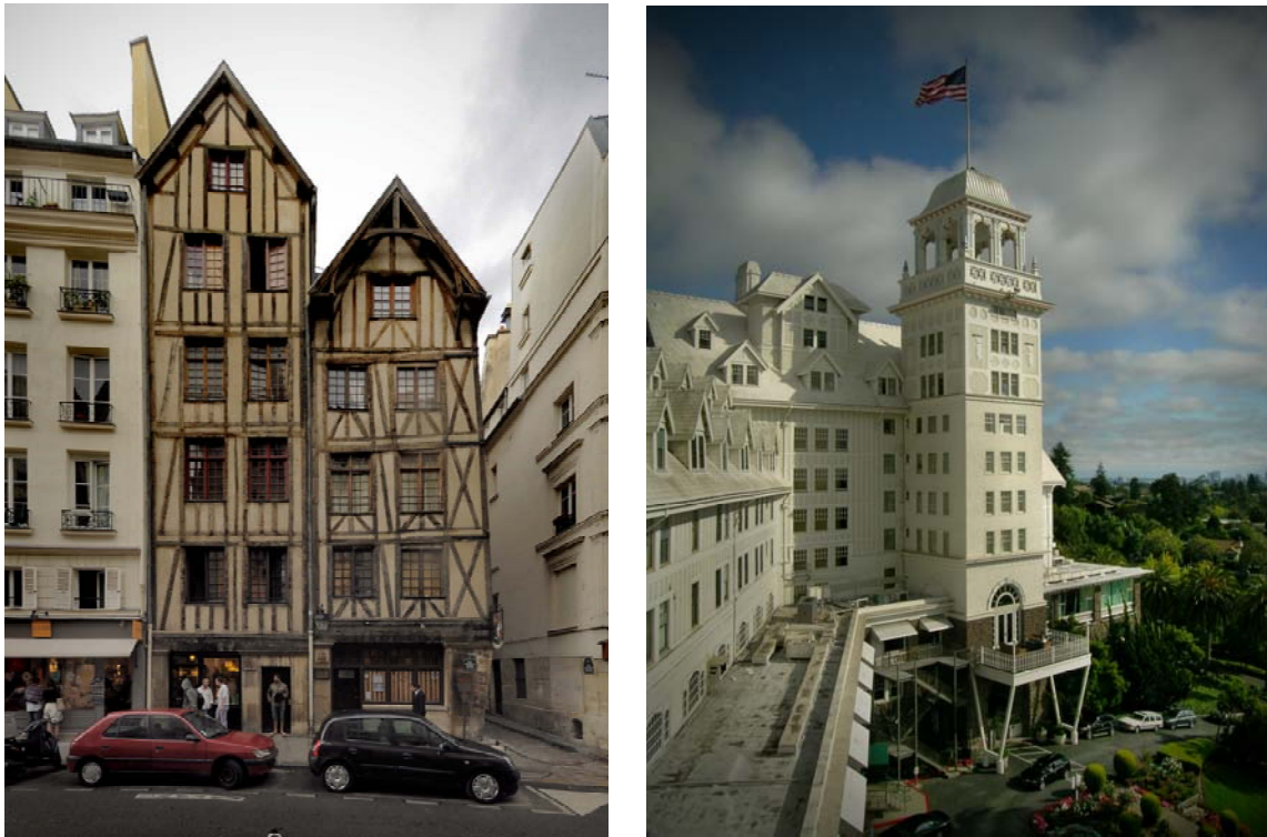
Figure 12&13: Left : Five and six storey Medieval houses in the Marais District of Paris, France, constructed beginning in the 14 th century, redone to their present form by the turn of the 16 th century, and restored in 1967, revealing the timber that had been plastered over. Right : The Claremont Hotel, constructed in 1906 in Oakland, California, USA has 11 storeys of occupancy in its tallest portion, including assembly spaces. The stone at the base is veneer onto the timber structure. Photos © Langenbach
