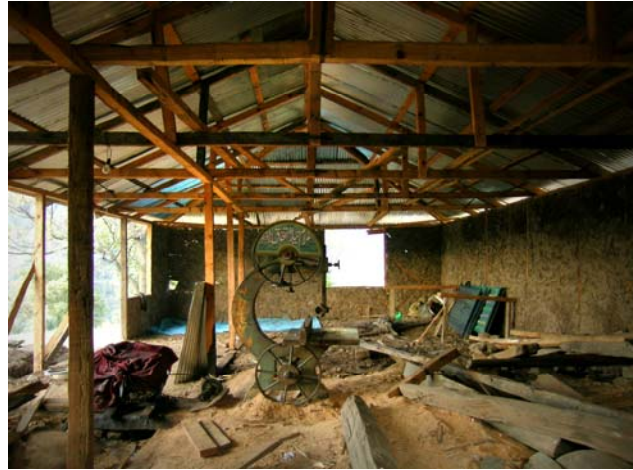
Figure 15&16: This dirt poor Pakistan Kashmir farmer who is rebuilding his house in the traditional dhajji dewari construction after the 2005 earthquake destroyed his rubble stone house. Not only is he doing the construction, but he is milling his own timber on the large old band saw visible in the photo of the interior on the right. Photos © Randolph Langenbach
