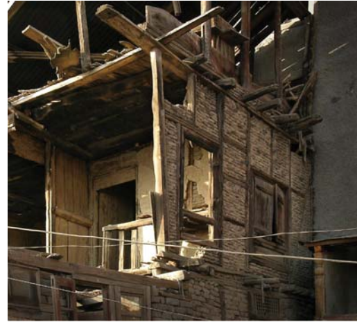
Figure 6&7: Left : Houses of traditional timber with mixture of timber-laced masonry (known locally as taq ) and timber frame with infill masonry construction, (known locally as dhajji dewari or “patchquilt wall” in old Persian) in Srinagar, Kashmir. Right : Partial demolition of dhajji dewari house reveals the timber frame and thin masonry wall construction. Photos © Randolph Langenbach.
