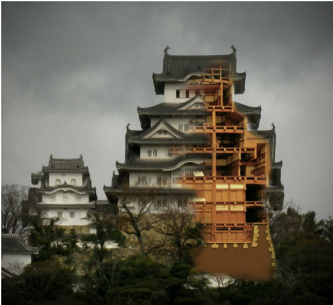
Figure 1: Seven-story timber frame Himeji Castle, Japan, 1608AD, overlaid with photo of model of interior timber frame structure. Photos and overlay © Randolph Langenbach.
