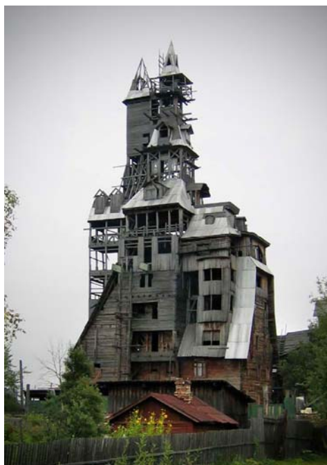
Figure 14: The 13 storey, 44 meter high single-family house constructed by Nikolai Sutyagin for himself and his wife in Arkhangelsk, Russia. It was never completed before it was demolished in 2009. Photo taken in 2004 by © Yury Kiselev, Panoramio.com
