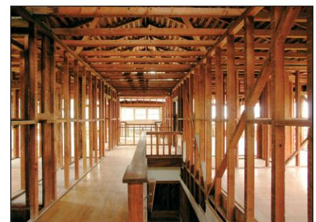
Fig. 3: Typical stud-frame of an early twentieth century house in California
