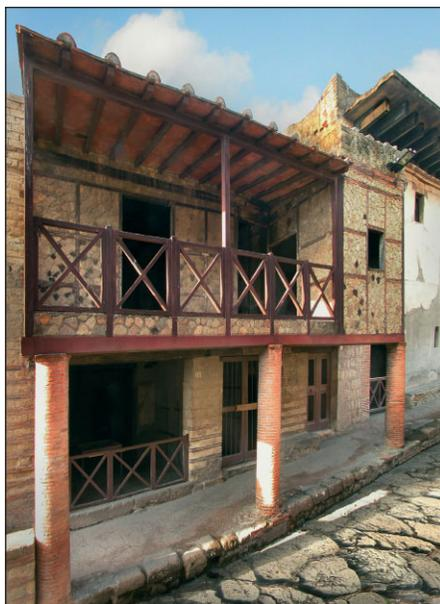
Fig. 4: Infill-frame house unearthed in the archaeological site of Herculaneum, Italy after being buried in the eruption of Vesuvius in 79 A.D.
