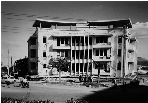
(a) Exterior of partially collapsed building after the 1965 San Salvador earthquake.
