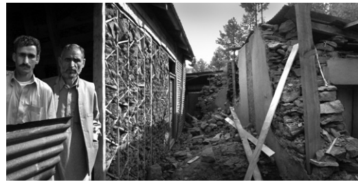
Fig. 5. Pakistan 2005, the carpenter and owner standing in their new dhajji dewari home to replace rubble stone house. The Pakistani government initially refused assistance for rebuilding with timber-laced masonry, but later accepted and promoted this kind of construction.
