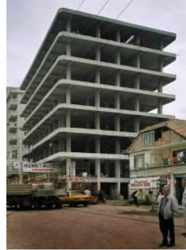
Figure 23: A massive RC frame in Golcuk, Turkey under construction at time of 1999 earthquake before installation of infill masonry walls. Much greater damage or collapse would have been likely had the infill walls been installed by the time of the earthquake.
