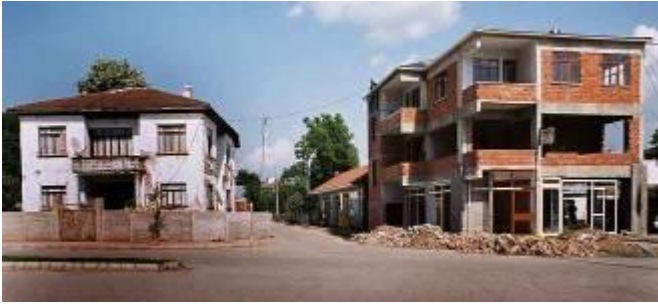
Figure 29: Three story RC building next to a 2½ story hımış house near Düzce after the 1999 Düzce earthquake showing the repair of severe damage to the RC building (notice the size of the ground floor columns). The hımış structure has lost only stucco on the side. Almost all of the hollow clay block on the RC building has been reconstructed after the earthquake. This shows that even low rise RC buildings sometimes suffered more damage than nearby traditional buildings.
