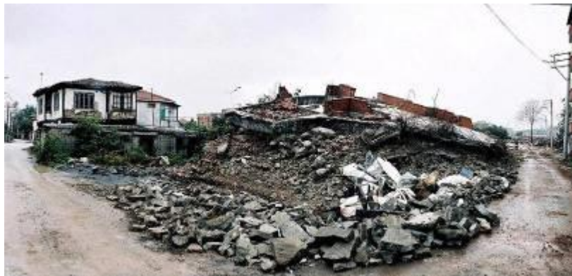
Figure 4: Surviving hımiş house next to a row of collapsed reinforced concrete buildings, Adapazari, Turkey, 1999.
