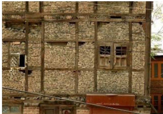
Figure 14: Example of Dhajji Dewari construction in Srinagar, 2005. The timbers form a complete frame, and the masonry is inset into the frame.
