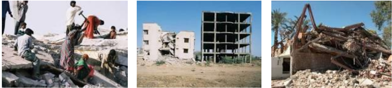
Figure 5: Demolition workers on collapsed RC infill building in Bhuj, 2001 one month after the Gujarat Earthquake. Women work alongside men in heavy construction tasks in India.
