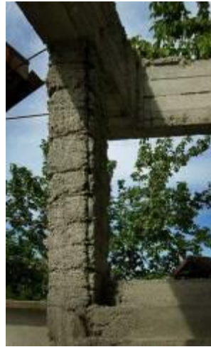
Figure 8: LEFT: House being reconstructed to replace one destroyed in Afyon earthquake. Concrete is being mixed on ground with garden hose and without slump test or measurements.
