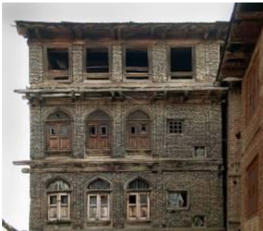
Figure 13: Example of Taq construction in Srinagar, Kashmir, 2005. The timbers in the masonry walls only run horizontally parallel to the wall and through the wall.
