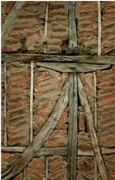
Figure 1: Detail of traditional hımiş construction in Turkey in mid-20 th century house in Gölcük.
