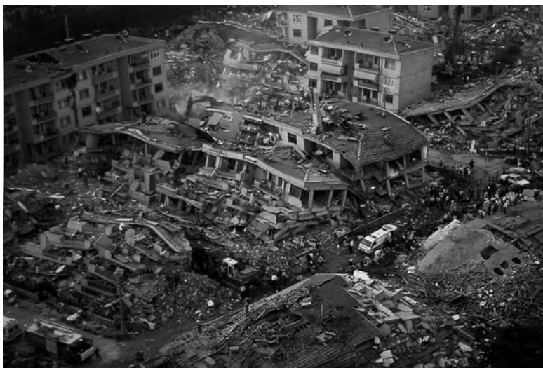
Fig. 3 Aerial view of collapsed apartment blocks, Gölçük (photo courtesy UN-ISDR)
