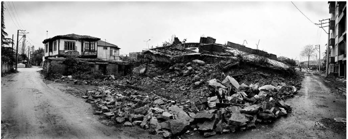
Fig. 4 Surviving humiş house next to a row of collapsed reinforced concrete buildings, Adapazari, Turkey, 1999 (photograph © Randolph Langenbach)
