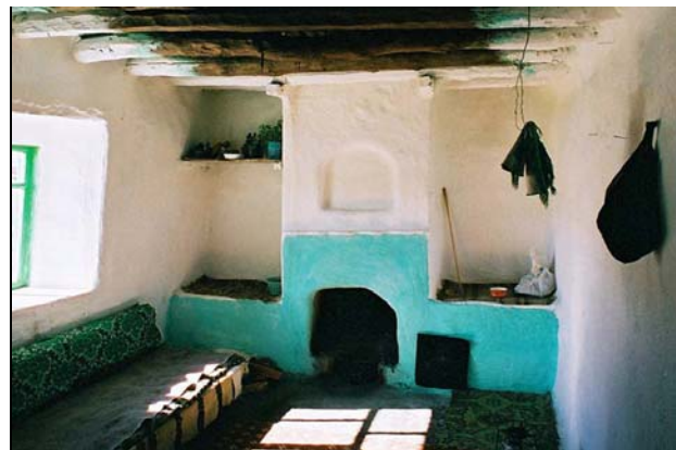
The same room photographed a year after the earthquake after the family had repaired and moved back into the traditional farm dwelling.
