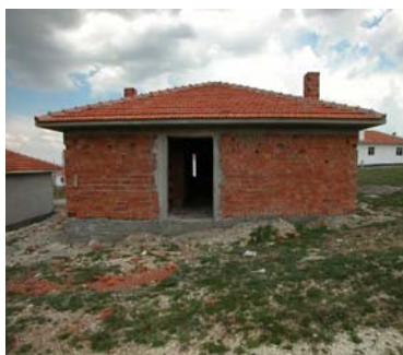
New house at a remote site constructed to re-house residents of Yuva – constructed of unreinforced hollow block masonry.
