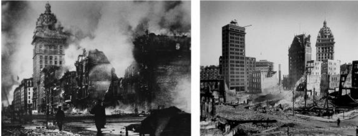
Figure 7. San Francisco in 1906 showing Chicago Frame buildings that burned out but remained standing. All of the taller buildings in these images are still extant in 2006. (Bancroft Library)
