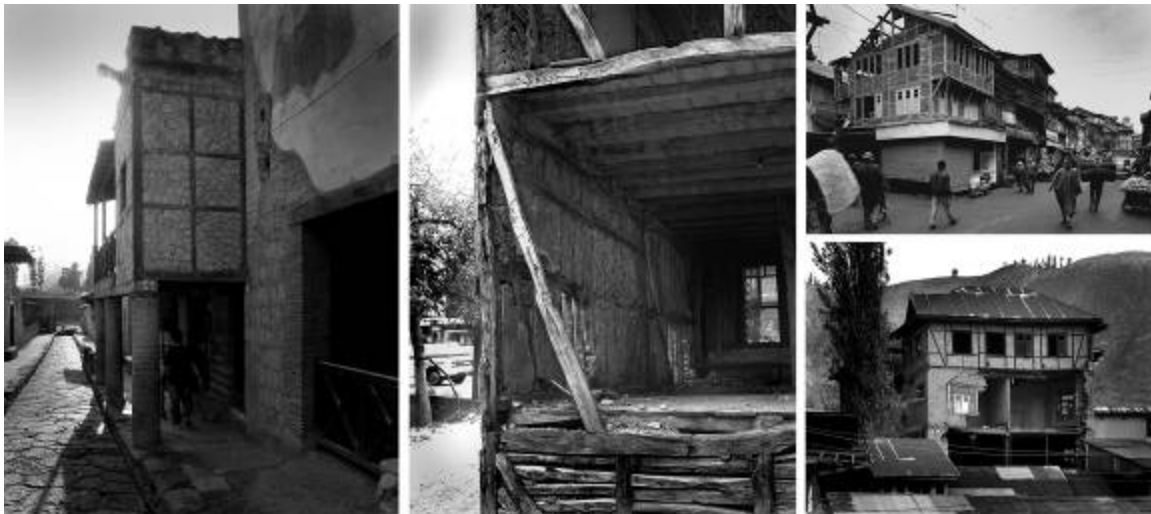
Figure 15. (L) Herculaneum “ Craticii ” construction. (C) Himis Construction, Turkey. (R) New Dhajji Dewari construction, Srinagar, in 1981, and house in Baramula after 2005 Kashmir earthquake.
