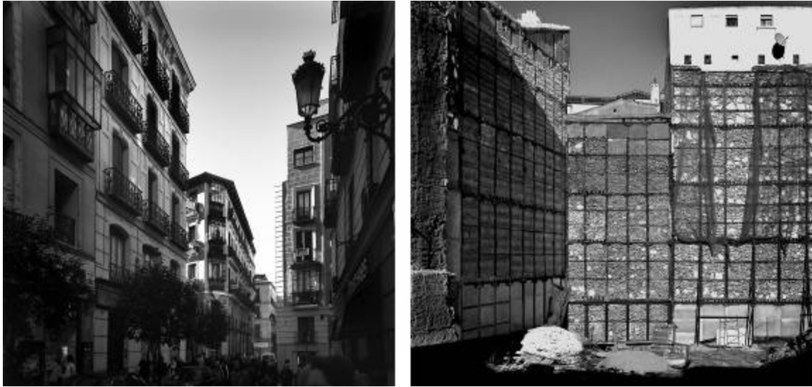
Figure 12. Historical center, Madrid showing front façades and infill masonry timber frame construction revealed on rear walls after demolition of adjacent structures in 2002.
