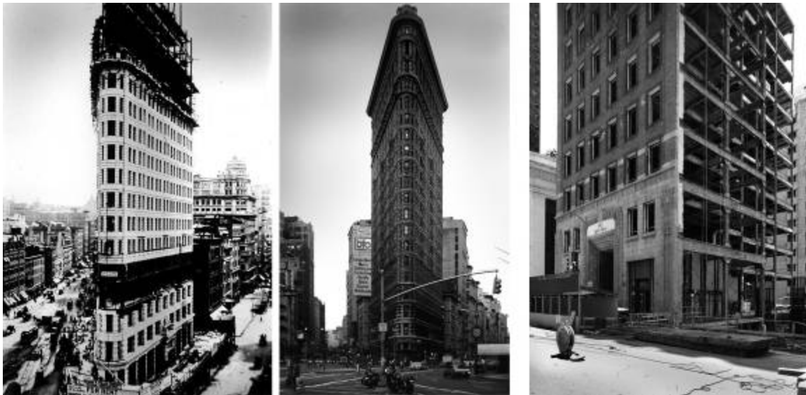
Figure 4. (L) Flatiron Bldg (1902), NYC. Masonry façade with construction beginning on upper floors at same time as at foundation (vazyvite.com). (C) Flatiron Bldg. (R) 343 Sansome, San Francisco.
