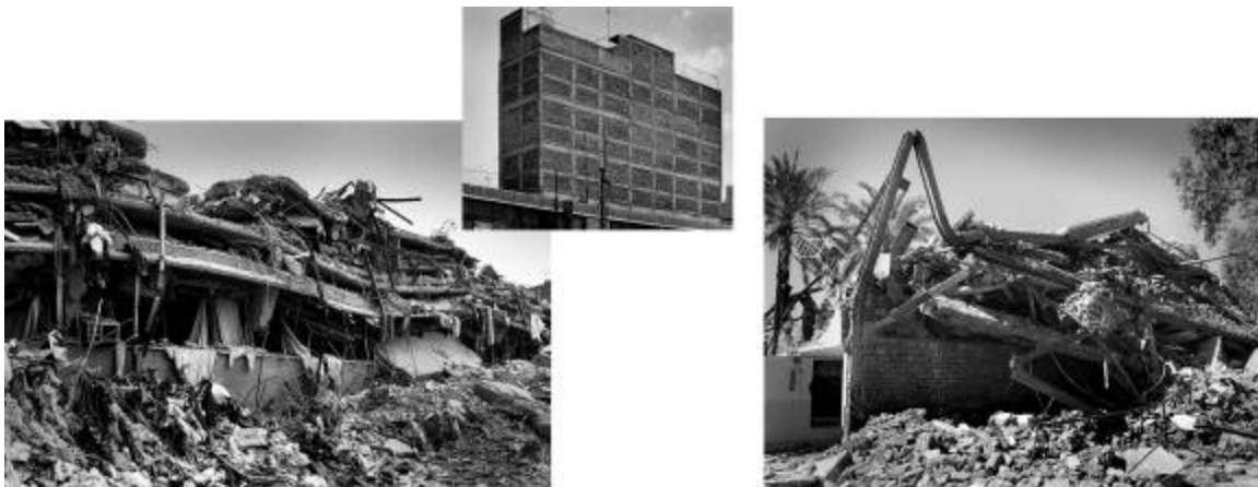
Figure 2. (L) Juarez Hospital after 1985 Mexico City earthquake with neighboring (C) undamaged infill-frame RC building. (R) Steel building after 2003 Bam, Iran earthquake.
