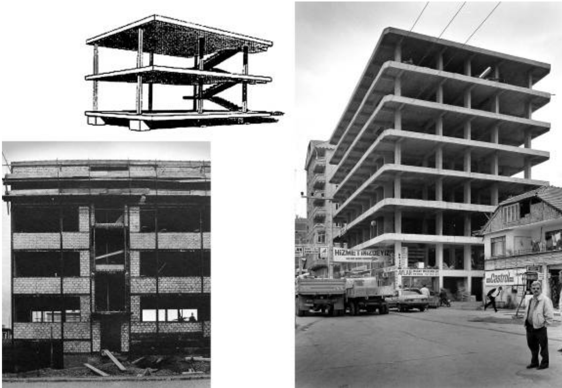
Figure 10. (L) Construction in 1927 of Stuttgart Werkbundsiedlung (Giedion, 1928). (C) Le Corbusier’s Dom-ino House, 1915. (R) Gölcük, Turkey building under construction at time of 1999 earthquakes.
