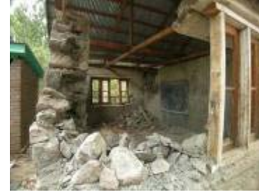
Figure 27: Detail of rubble masonry construction of school building seen on left in Figure 26.
