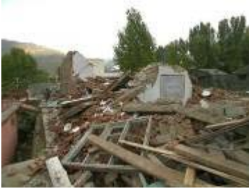
Figure 25: Totally collapsed unreinforced masonry school building in Uri Government Complex.
