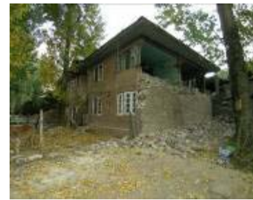
Figure 30: Brick building with rubble stone end walls in Uri Government complex.
