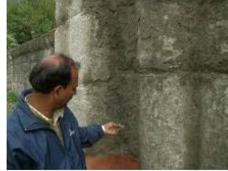
Figure 19: Leaning column. Bell chain shows vertical line.
