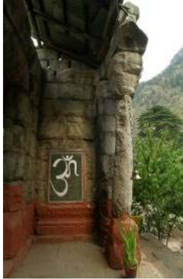
Figure 19: Leaning column. Bell chain shows vertical line.
