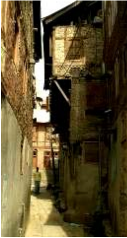
Figure 11: Narrow lane in Baramula Old City with Dhajji Dewari top floor construction.
