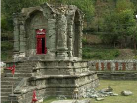
Figure 21: Detha Mandir Temple showing stones thrown off from the top of the wall. It appears that unconsolidated and deteriorated stone work surrounded a later reinforced concrete roof, which is set back from the edge of the structure. Differences in the vibrations between the roof and surrounding stonework may have contributed to the damage.
