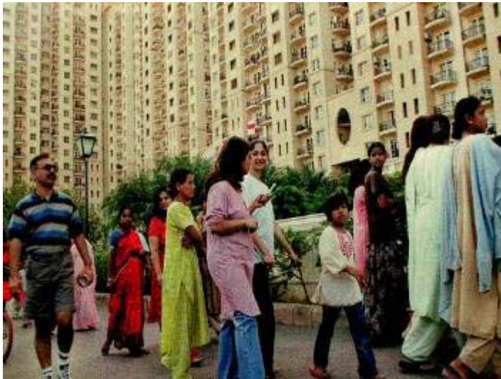
Figure 2: Gurgaon highrise during evacuation (photo from India Today )
