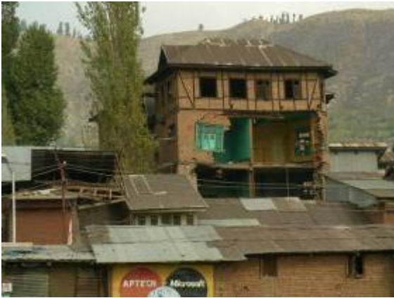
Figure 9: Large house in Baramula showing collapse of URM wall, leaving Dhajji Dewari construction wall in place above.
