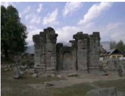
Figure 14: Shiva Temple, Fatehgarh. Stones in Fig.15 show some shifting from earthquake.
