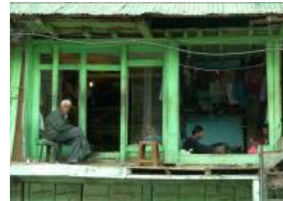
Figure 35: In Uri, this and many other shops were open and in active use in wooden buildings, or even some partially damaged masonry buildings.
