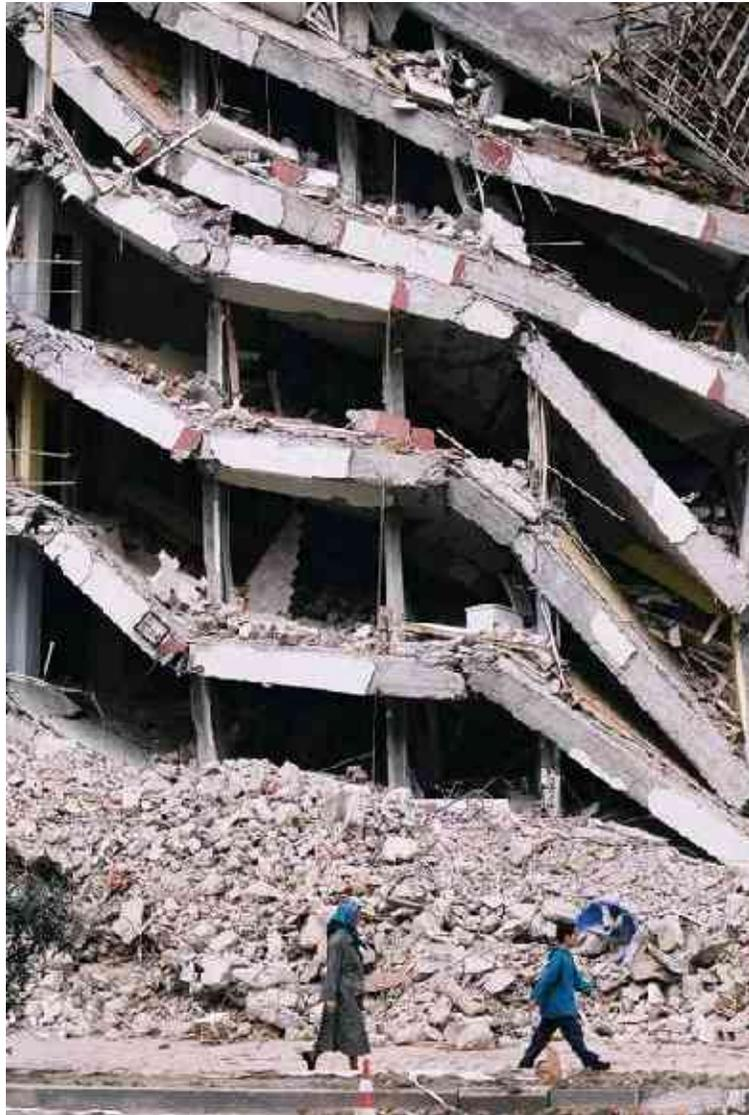
Figure 15: Collapsed Reinforced concrete building in Gölcük.
