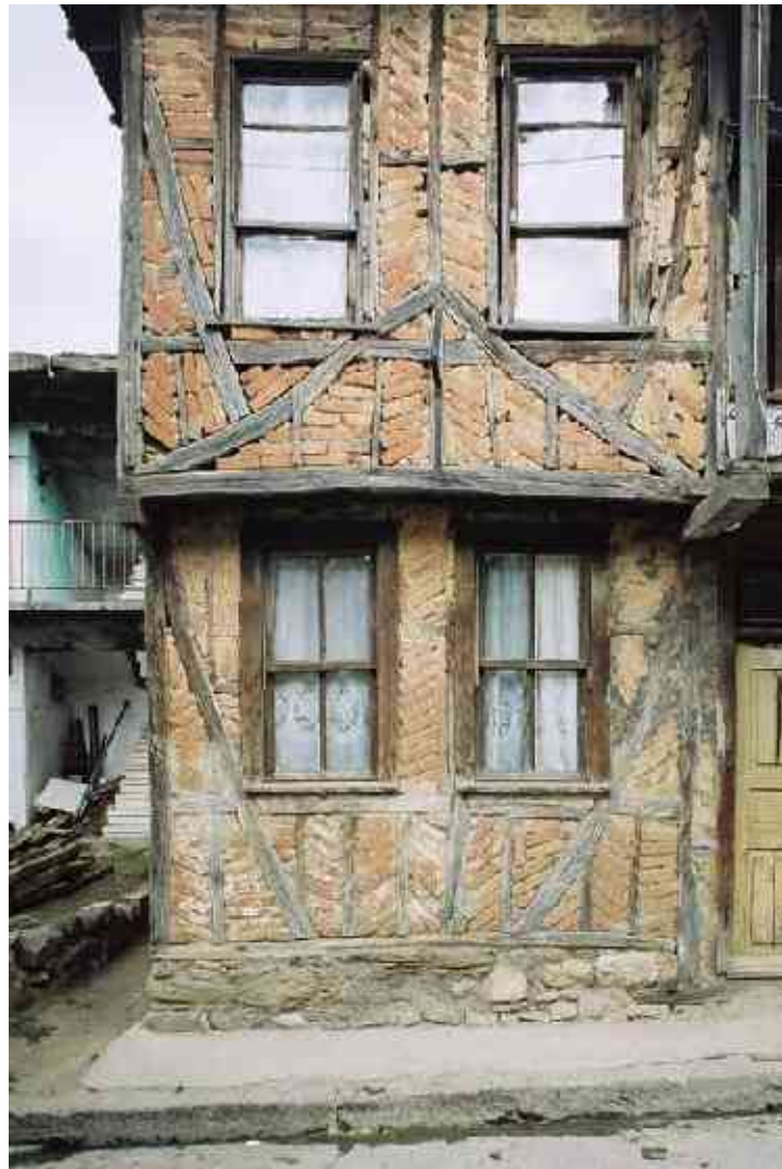
Figure 11: Hımış house in Gölcük after earthquake constructed in 1955. There was only slight damage to the interior of this house.
