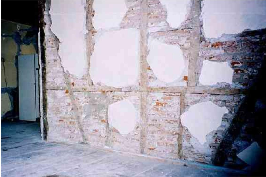
Figure 12: *Hımış* interior wall in Düzce after earthquake.
