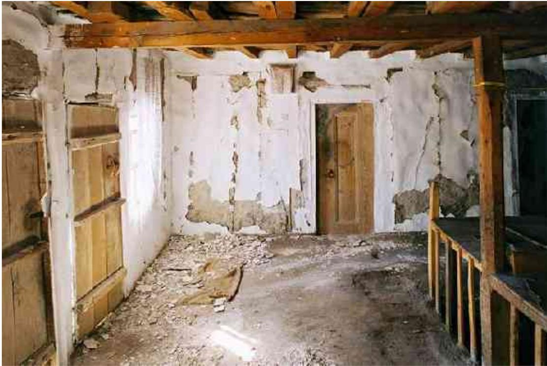
Figure 13: Interior of *hımiş* house in Orta after earthquake showing damage to mud and lime plaster over infill walls.
