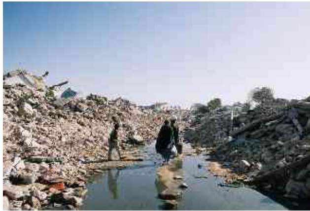
Figure 1: View of Anjar City Center after the Bhuj Earthquake of January 26, 2001.
