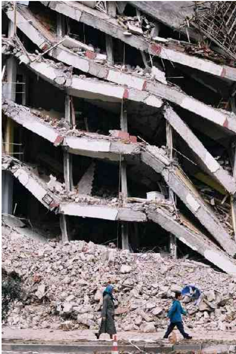
Figure 15: Collapsed Reinforced concrete building in Gölcük.
