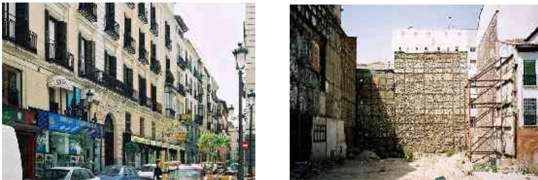
Figure 2 a&b: Timber and masonry infill-frame construction near the Plaza Major in Madrid – hidden in the facades, but revealed by demolition behind.
