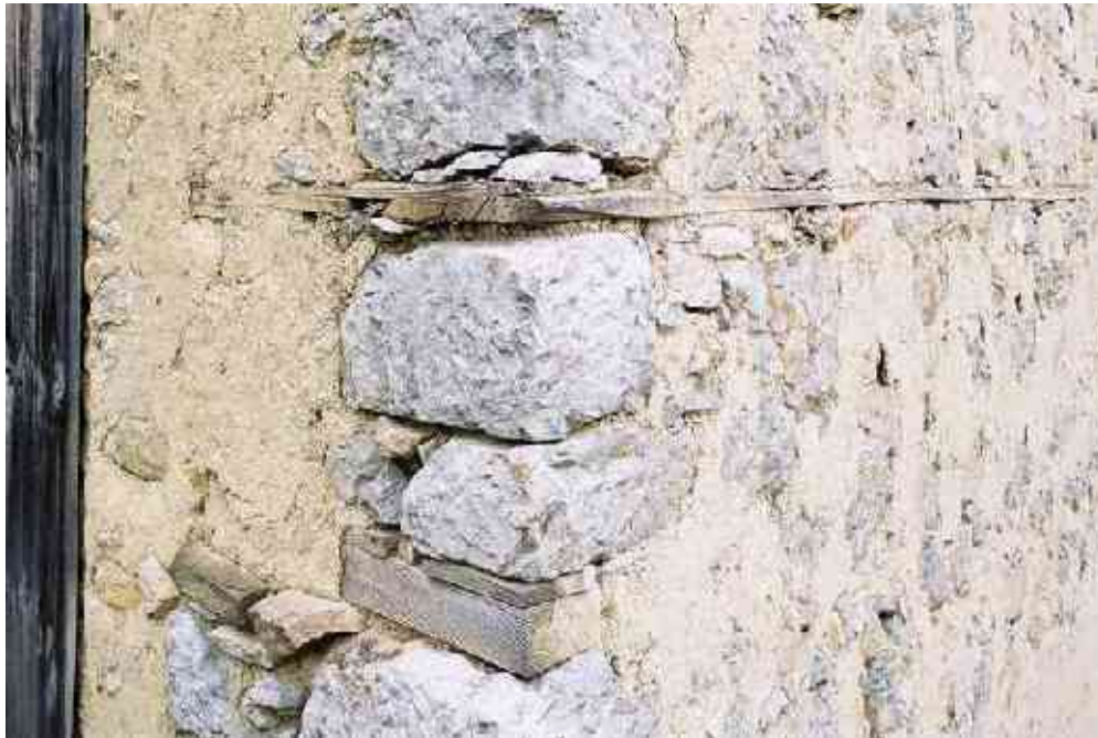
Figure 10: Laced bearing wall in Safranbolu, Turkey
