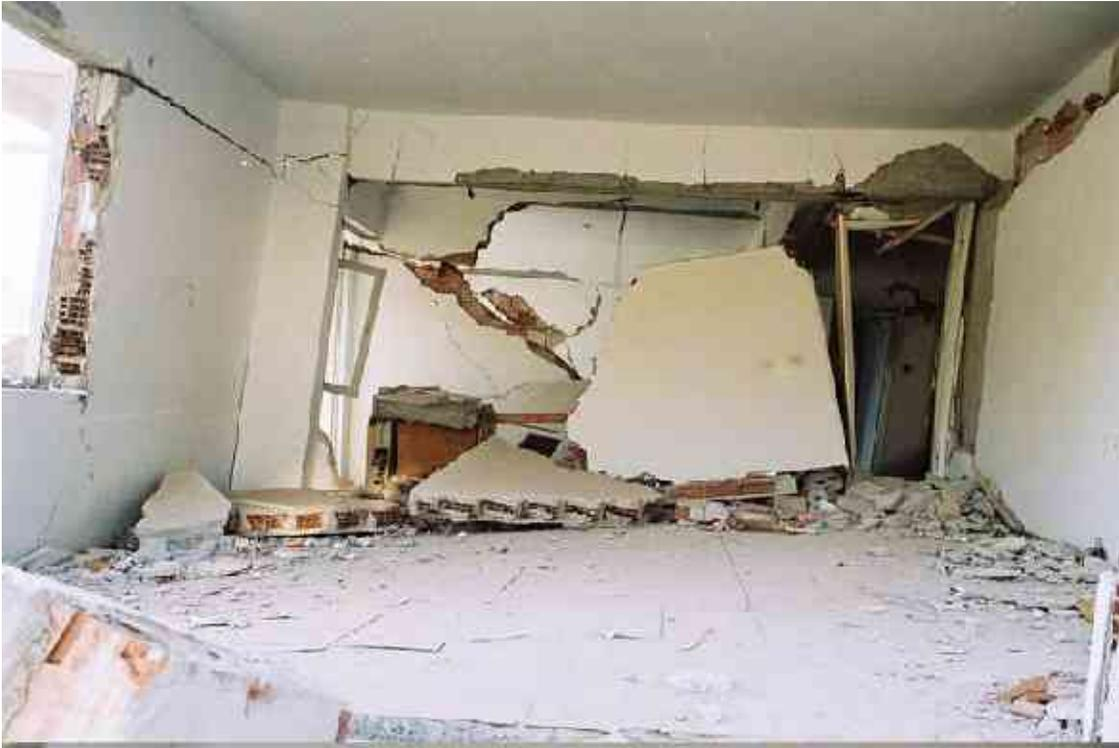
Figure 14: Collapsed interior infill wall in reinforced concrete building in Gölcük
