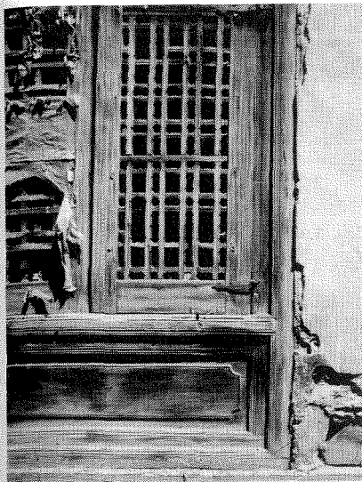
The Jalli shutters showing, on the left, the remains of the paper attached for winter protection.
