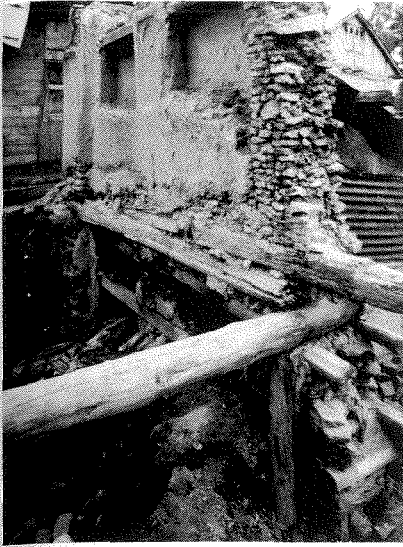
Above: A house in ruins shows the timbers imbedded at each floor level in the Taq System masonry wall.
