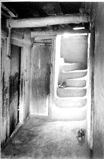
The entrance lobby of a typical traditional house showing the timber and mud interior finishes. This front lobby, located at the center of the house, is considered to be the safest place to go to during an earthquake. (Running out of the house is more dangerous.)
