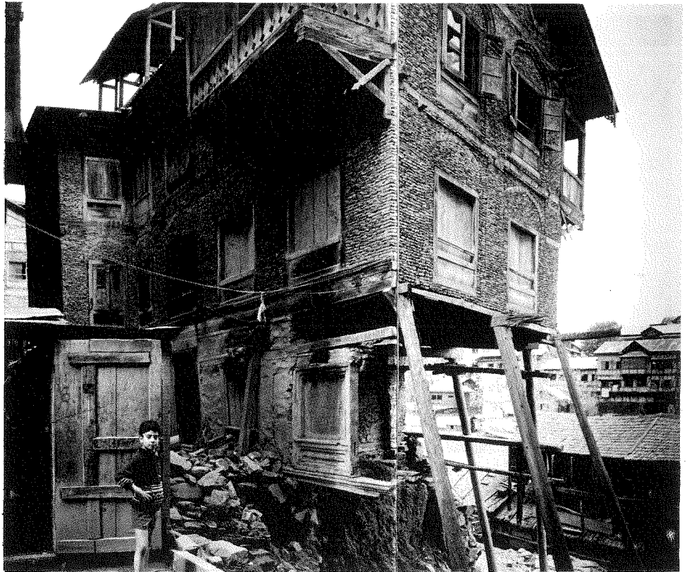
Above: A house in ruins shows the timbers imbedded at each floor level in the Taq System masonry wall.
