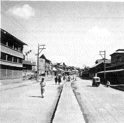
The new road constructed during the 1970's which replaced the picturesque 14th century Mar Canal which used to penetrate the heart of Srinagar. The sewerage line which was supposed to replace the canal was deleted in a budget cut, so now the sewerage which used to flow out of the city through the canal now backs up into Dal Lake.
