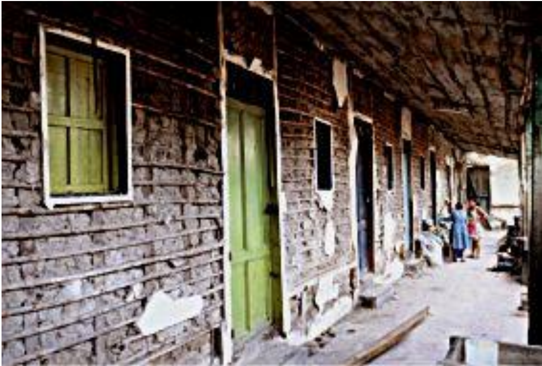
An example of BAHAREQUE construction, a native method in El Salvador, this building withstood the quake with little damage apart from plaster falling off the walls.
