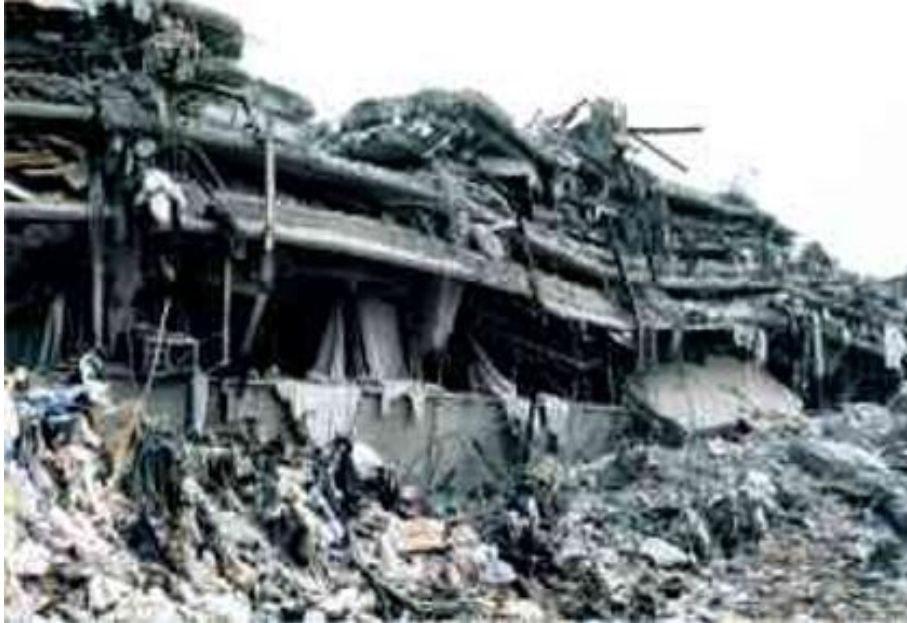
Collapsed building, Juarez Hospital, Mexico City, 1995
