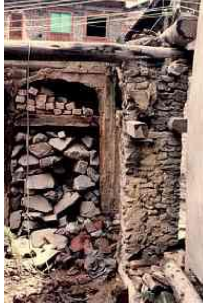
Srinagar House being demolished showing the Tag timber and masonry construction with timbers imbedded into the wall lengthwise and cross-wise.
