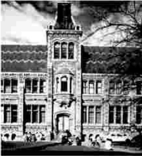
This building in New Zealand was strengthened by cables wrapped around the masonry structure. The cables function similarly to the runners in the TAQ system.
