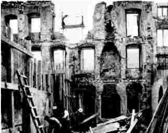
After the 1979 earthquake in Kotor Yugoslavia many buildings were completely gutted. Although the historic masonry was reattached the historic interiors have been completely destroyed
