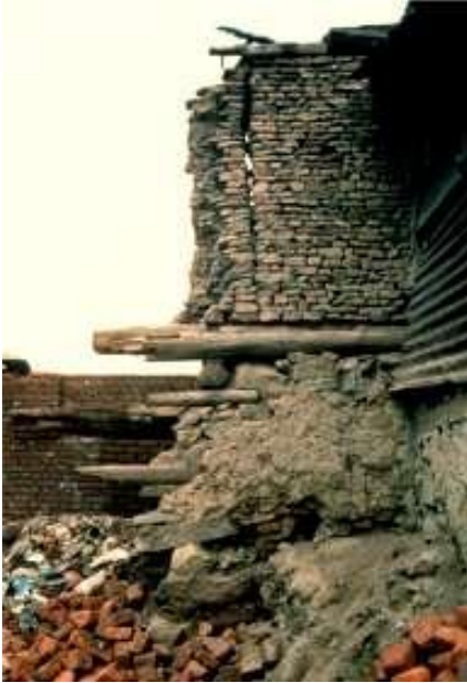
Srinagar House being demolished showing the Tag timber and masonry construction with timbers imbedded into the wall lengthwise and cross-wise.
