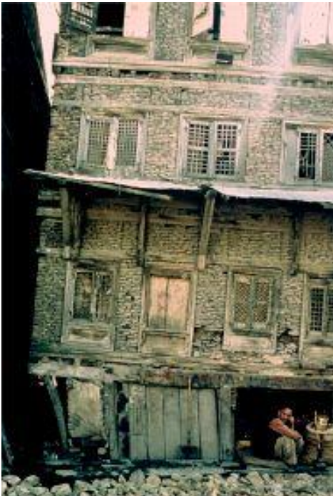
An eighteenth or early nineteenth-century canal warehouse in Srinagar illustrates the TAQ system of construction. The alternating timber "runners" and brick infill create a "woven" appearance.
