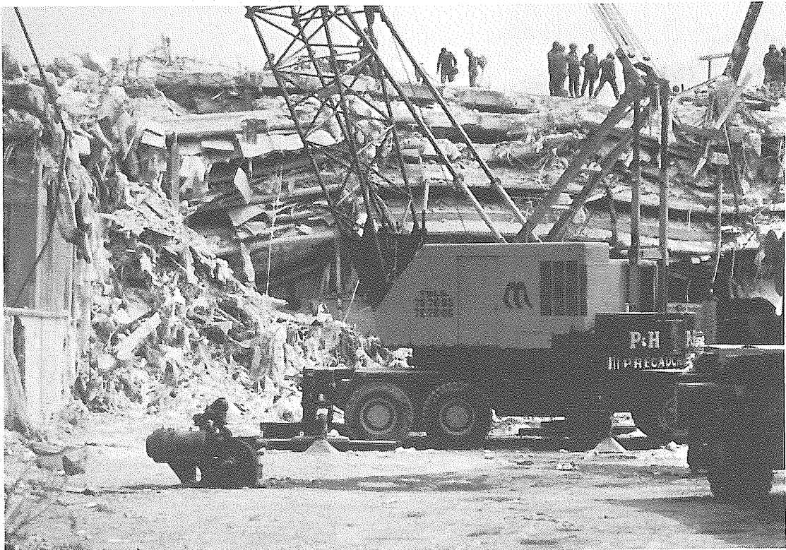
9. MEXICO CITY, pancake collapse of a reinforced concrete column and waffle structure.
